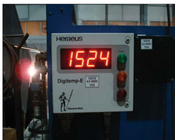
Fig. 16: Dip temperature unit.
